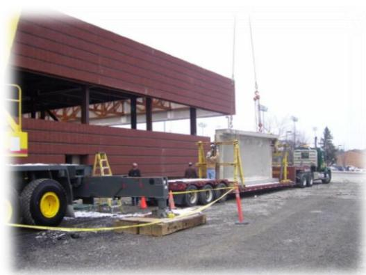
**Figure 2: Precast Panel Site Delivery & Installation**
